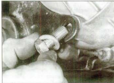
8.15a Unscrew the two bolts securing the rear mounting to the transmission . . .
